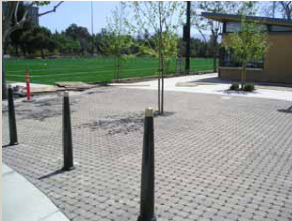
Permeable Pavers, Mayfield Playing Fields, Palo Alto
