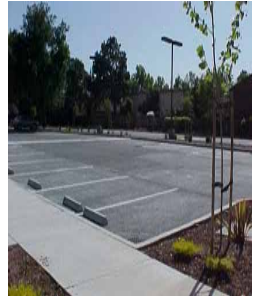
Pervious Concrete Parking Lot, Congregation Sinai, San Jose
