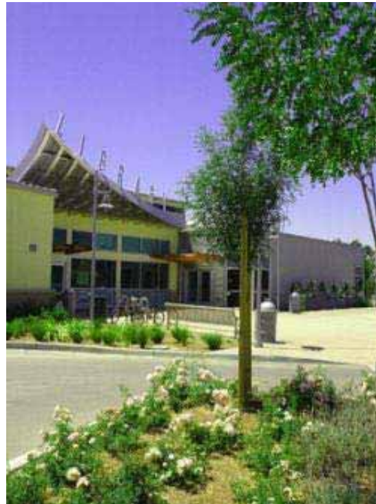
Vegetated Bioswale, Tully Library, San Jose
