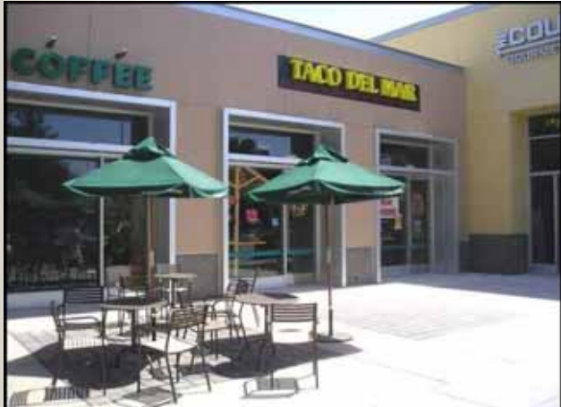
Pervious Paving, Starbucks/Taco del Mar, Palo Alto
