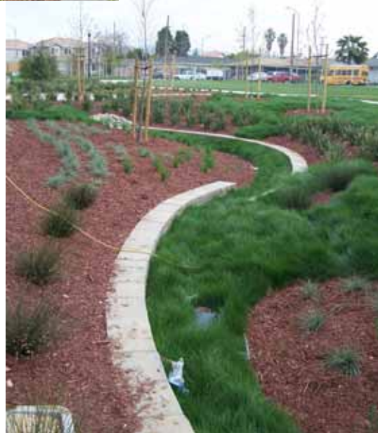
Vegetated Swale Integrated into Park Landscaping, Modern Ice, San Jose
