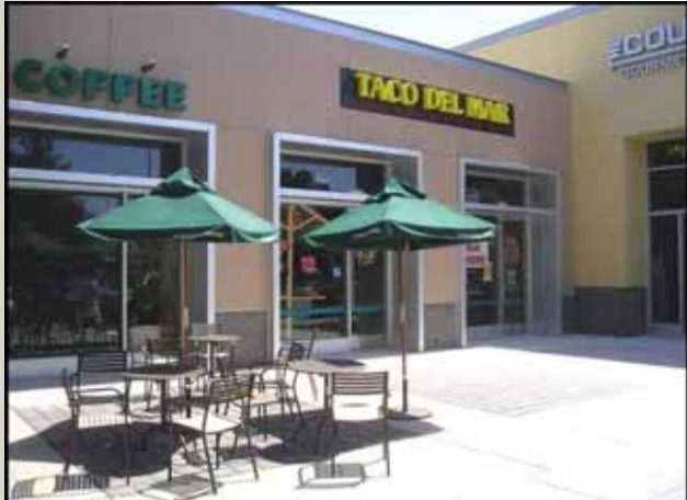
Pervious Paving, Starbucks/Taco del Mar, Palo Alto
