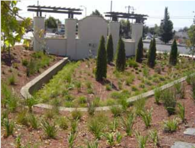
Vegetated Swale and Detention Area Behind Entrance Sign, Modern Ice, San Jose
