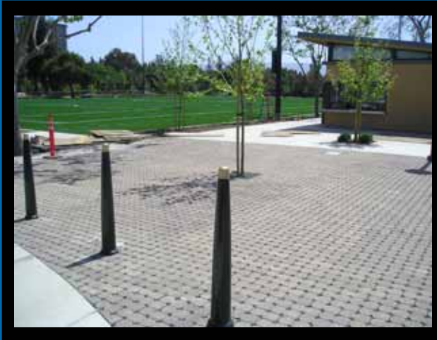
Permeable Pavers, Palo Alto/Stanford Community Playing Fields
