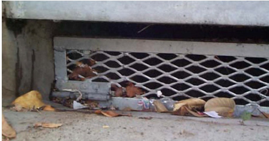
United Stormwater Screen Cover™ (courtesy of United Stormwater, Inc.).
