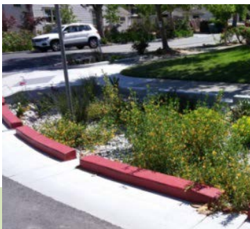
Biotreatment area in a curb bulb-out in the Southgate Neighborhood, Palo Alto
