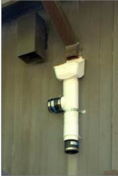
First flush and downspout diverter installation
