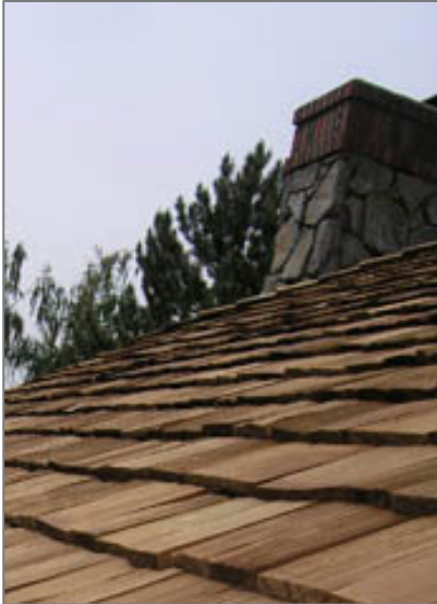
Wood shingle roof Courtesy of Gutter Glove
