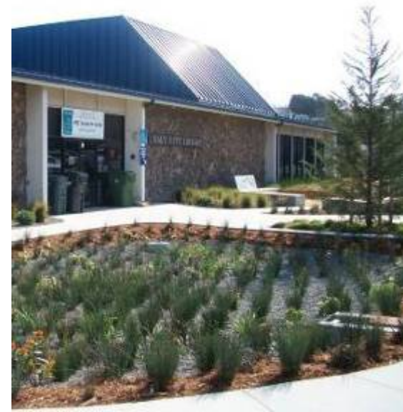
Bioretention Area, Serramonte Library, Daly City
