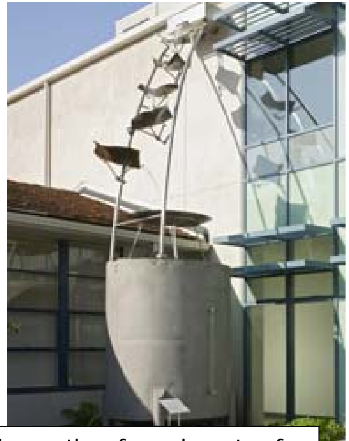
Harvesting for rainwater for indoor toilet flushing
