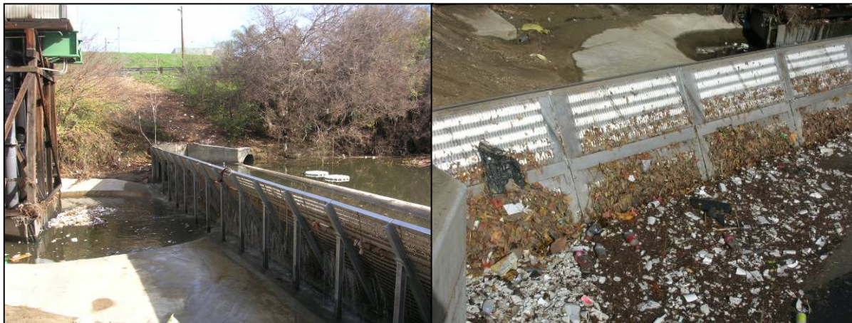
Photo 13- Inclined Louver Panel Screens within Caltrans Detention Basin, Pasadena, CA (Photo courtesy of Kevin McGillicuddy, Roscoe Moss Company, Los Angeles, CA)
