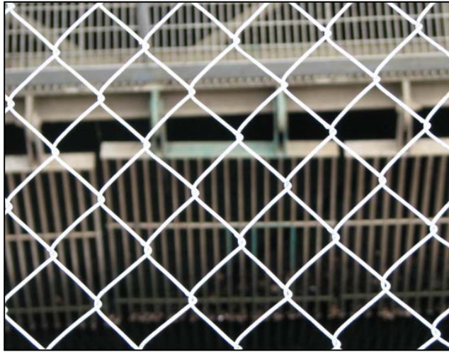
Photo 10 – Trash Racks at Intake to Oakmead Pump Station
