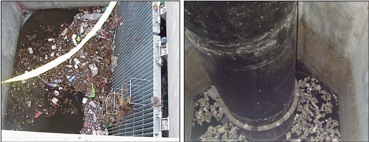
Photo 6 – (a) Trash rack and (b) Pump at the City of Santa Clara's Rambo Pump Station
