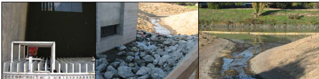
Photo 4 - San Francisquito Pump Station (a) Trash Rack; (b) Discharge Structure; and (c) Discharge Channel
