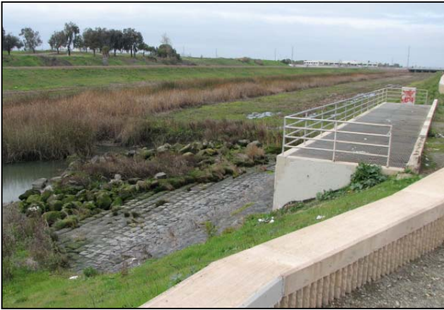
Photo 9 – Oakmead Pump Station Discharge Structure
