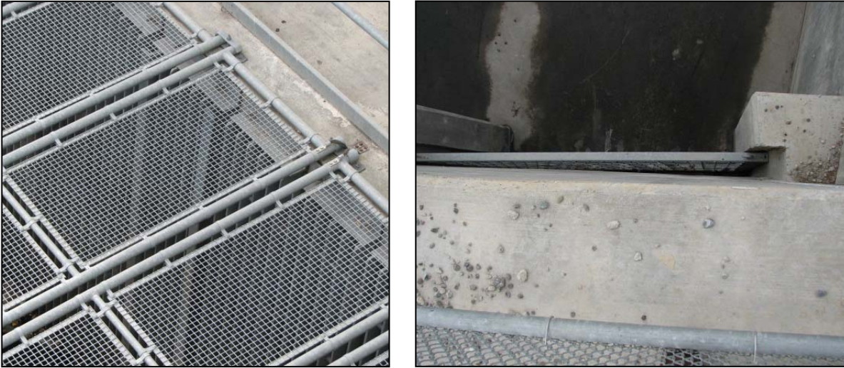
Photo 7 – Rincon 2 Pump Station Trash Management at (a) Intake; (b) Discharge
