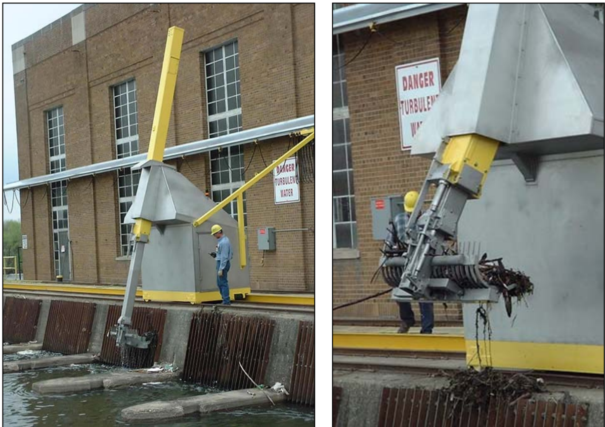
Photo 8 - Automatic Trash Rack Rake
