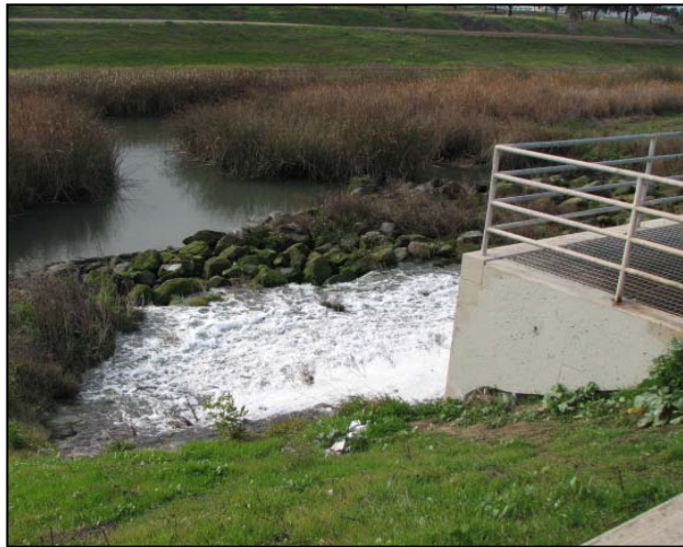
Photo 5- Water Flowing from Oakmead Pump Station
