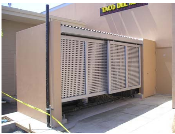
Covered trash enclosure reduces the potential for stormwater to come into contact with pollutants.
