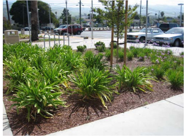
Vegetated bioswale at front of building collects runoff from surrounding walkways.
