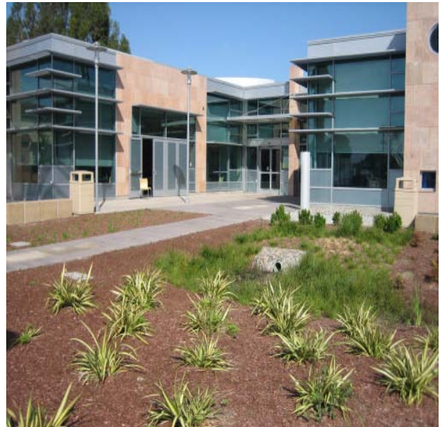
Roof runoff is directed to retention pond for natural treatment of stormwater.
