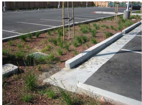
← and ↑ Curb cuts allow parking lot runoff to drain to vegetated bioswale.
