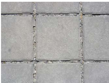
Close-up of permeable pavers.
