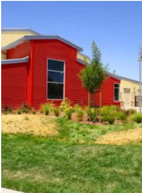
Vegetated bioswale collects runoff from building
