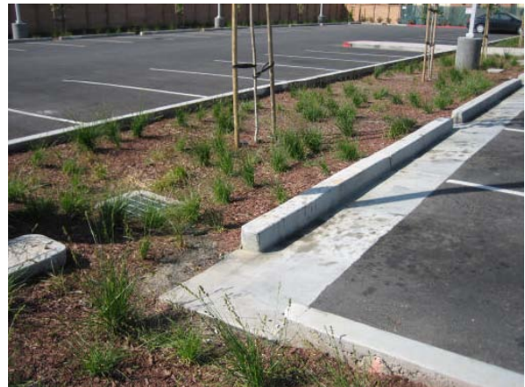
← and ↑ Curb cuts allow parking lot runoff to drain to vegetated bioswale.
