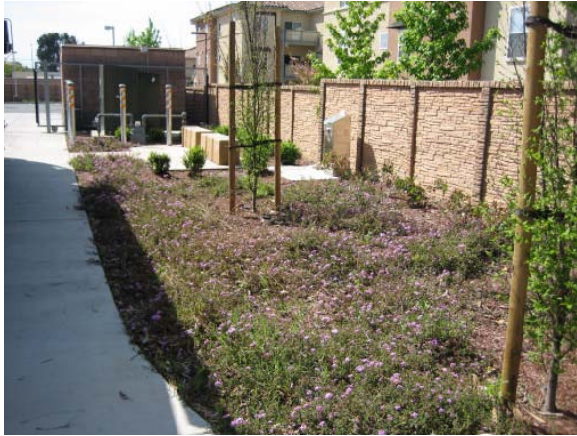
Vegetated bioswales at rear of building collect runoff from roof downspouts and walkway.
