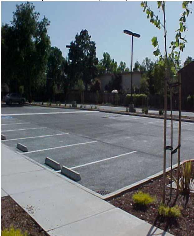
Pervious concrete parking lot reduces impervious surface and treats stormwater.
