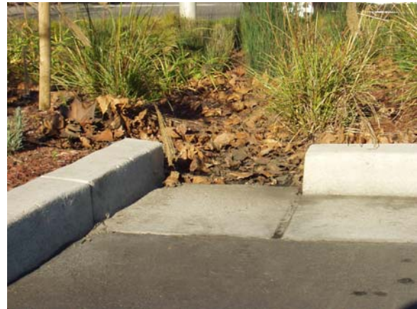
Close-up of curb cut leading to vegetated bioswale.
