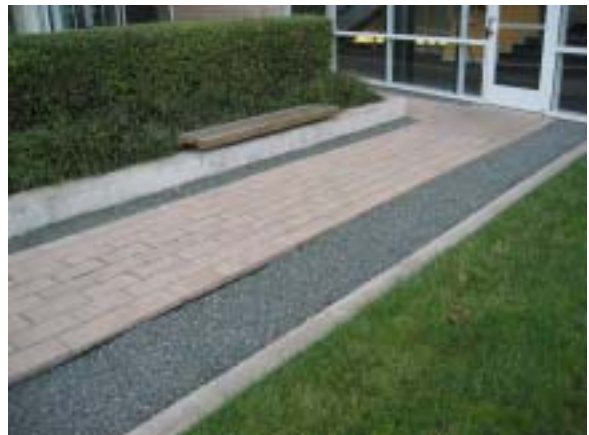
Turf and gravel surrounds this pathway, providing an area for infiltration to occur.
