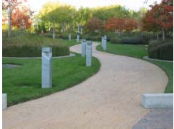
Permeable pavement and landscaped areas fill the courtyard on top of the parking structure.
