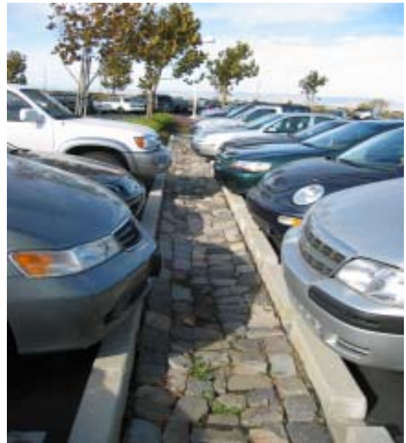
Rectangular stones are used to create a rocky swale.
