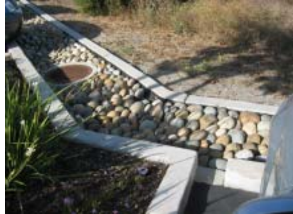
This rocky swale has a storm drain for excess flows.
