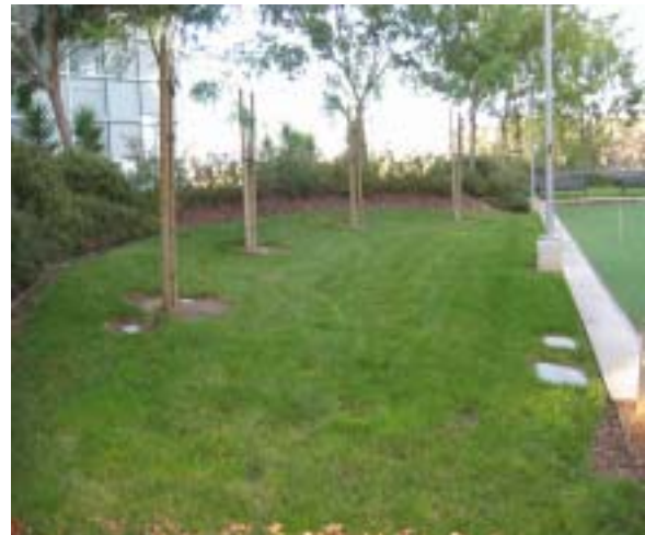
This grassy rooftop area planted with trees reduces and provides some natural treatment of runoff.
