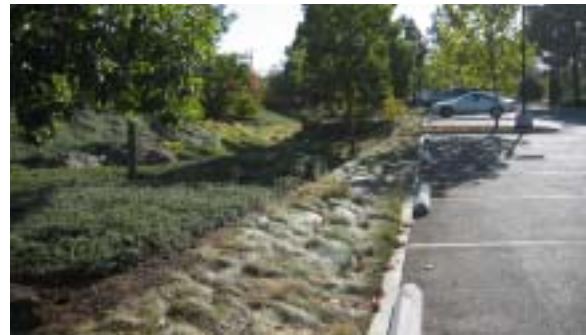
The detention basin collects water from the parking lot. The concrete edging protects the asphalt from water damage while the bumper stops help prevent cars from traveling over the vegetated swales.
