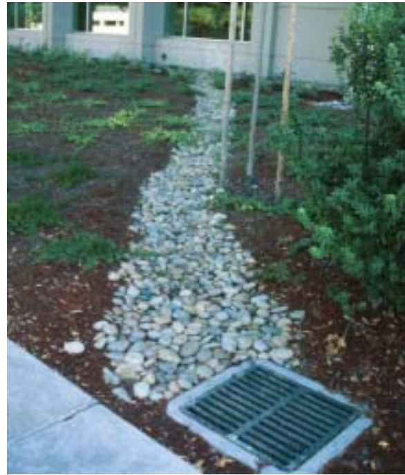
This rocky swale is used to slow and treat rooftop runoff before draining to the storm drain. A minimum two percent (2%) slope away from the building protects the building foundation from water damage.
