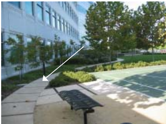
This pathway made of pervious pavers allows infiltration through the sand filled crevices. Also, these benches are provided on pervious surfaces.
