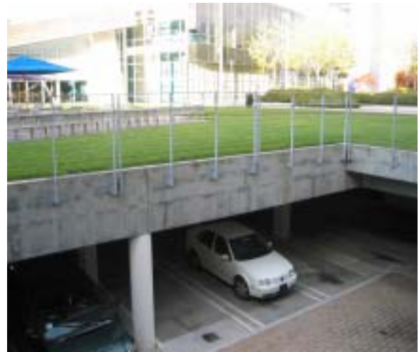
The parking lot can be seen below the turf on the level above.
