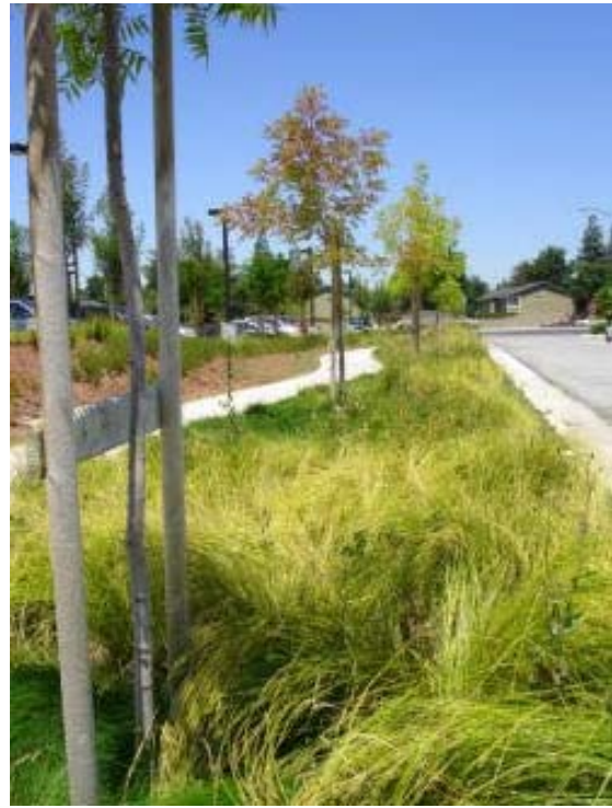
Carex grasses in vegetated bioswale
