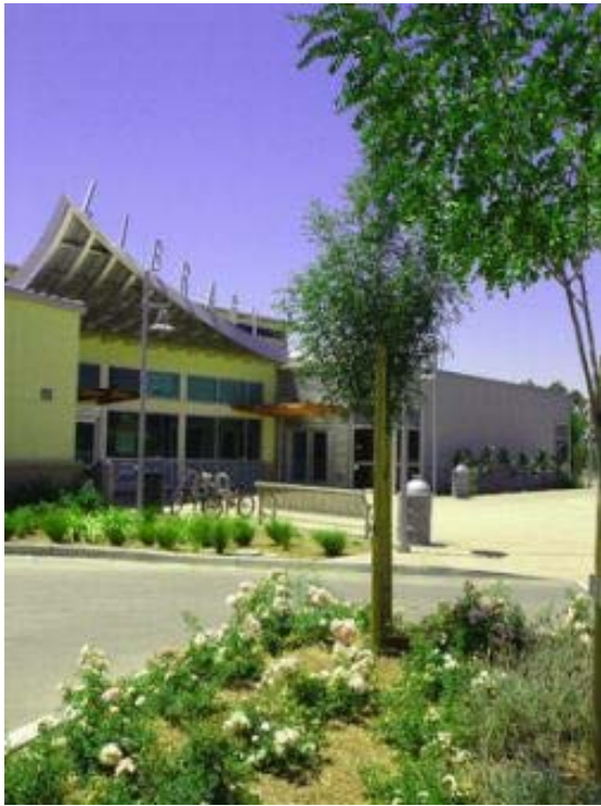
Runoff from parking lot drains to vegetated bioswale
