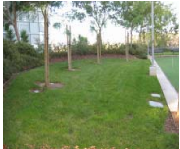
This grassy rooftop area planted with trees reduces and provides some natural treatment of runoff.
