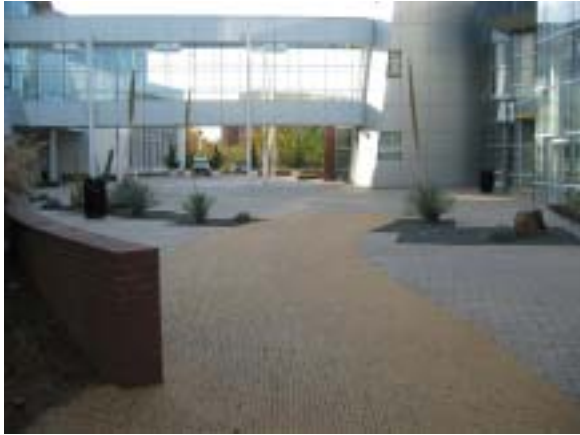
Permeable pavement is used in this courtyard.
