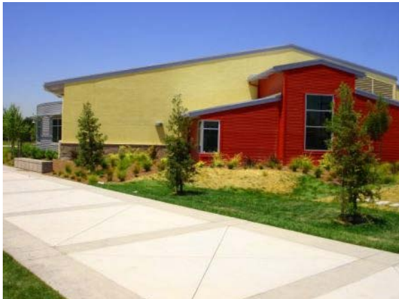
Vegetated bioswale collects runoff from walkways (above and right)
