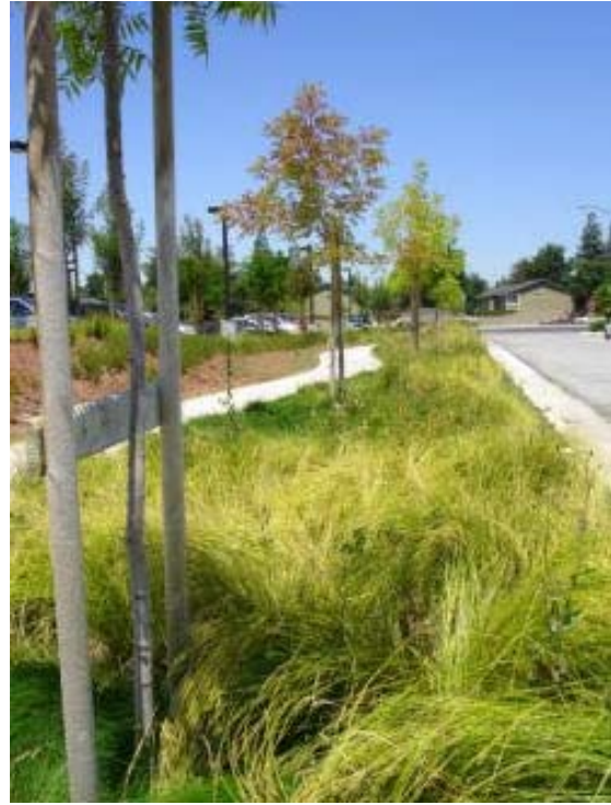
Carex grasses in vegetated bioswale
