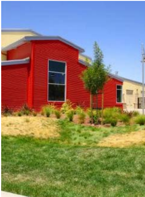
Vegetated bioswale collects runoff from building
