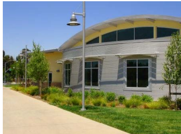
Walkway and roof runoff drain to vegetated bioswale
