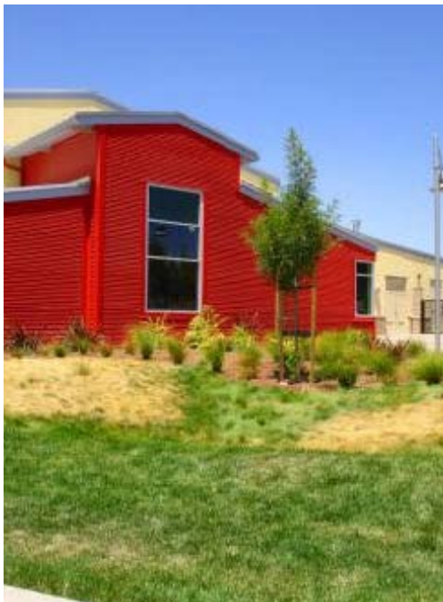
Vegetated bioswale collects runoff from building
